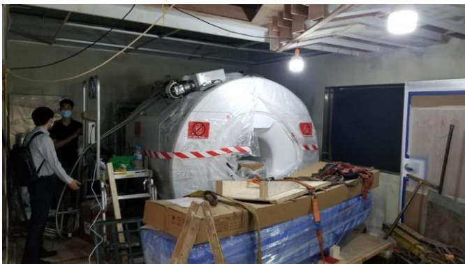
↑ MRI Done installation →
